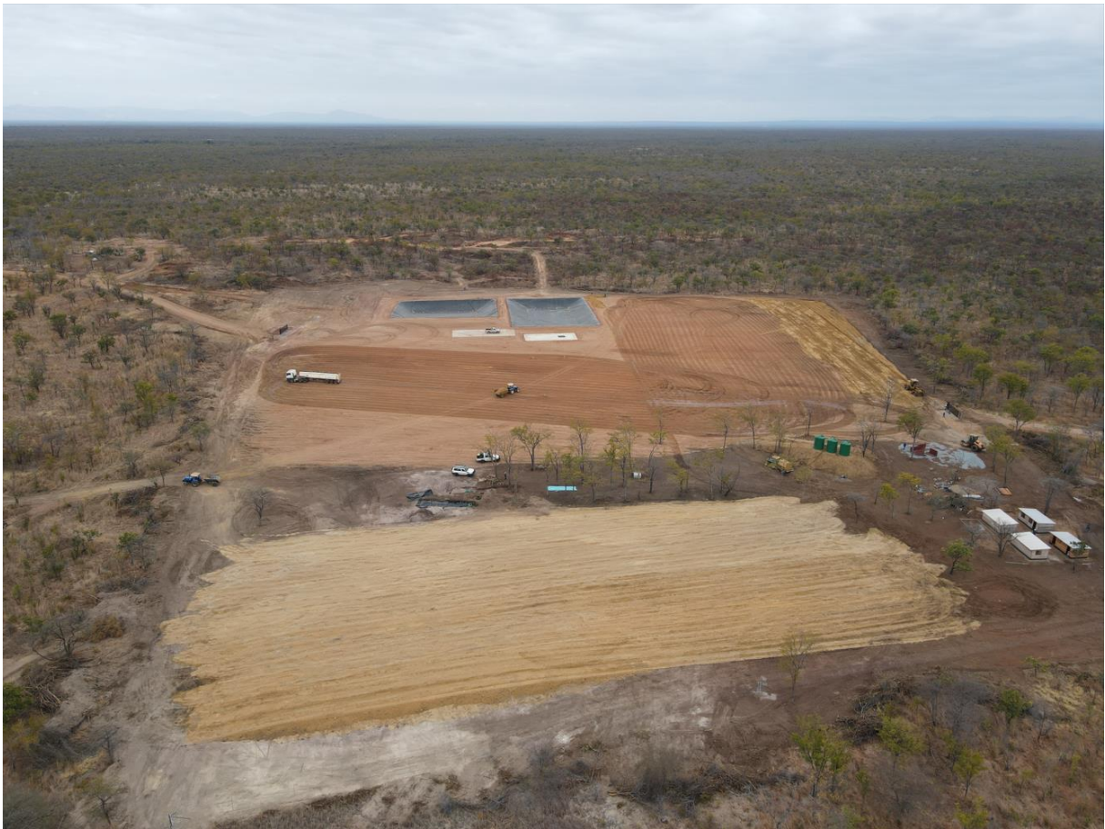
Figure 1 - Mukuyu-2 wellsite completed ahead of Rig 202 mobilisation
