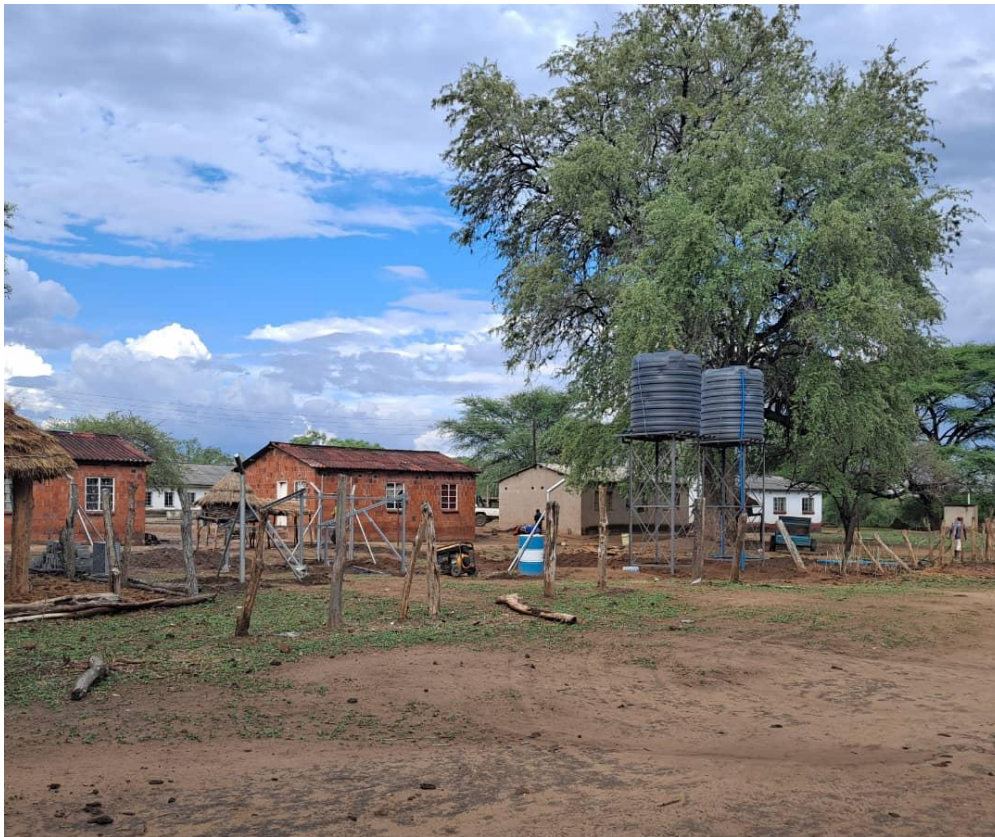
Figure 2 - Installation of permanent water supply to Masoma Clinic and School
