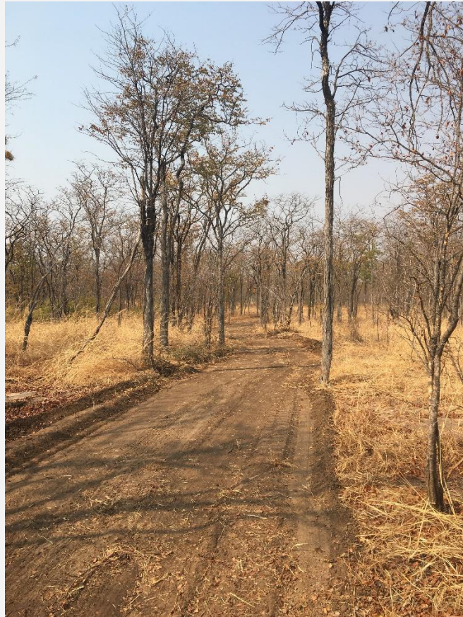
Figure 2 – Example of low impact seismic line clearing
